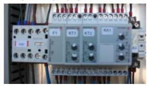
Verify that drive motor current limiter GAVAZZI DIB71 (KA1), located in control box on side of contactor (KM2), has the following setting.
